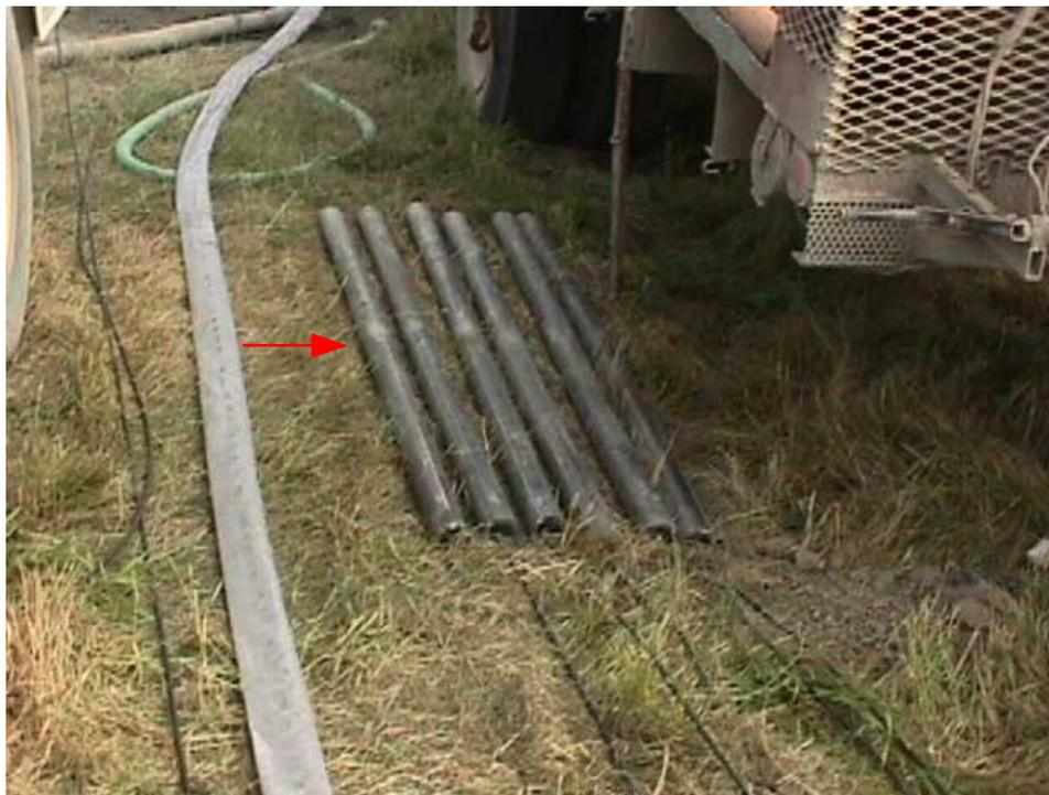
**Figure 4 - Center Tap Tubular HSCI Anodes. Cable to anode connection at arrow.**
